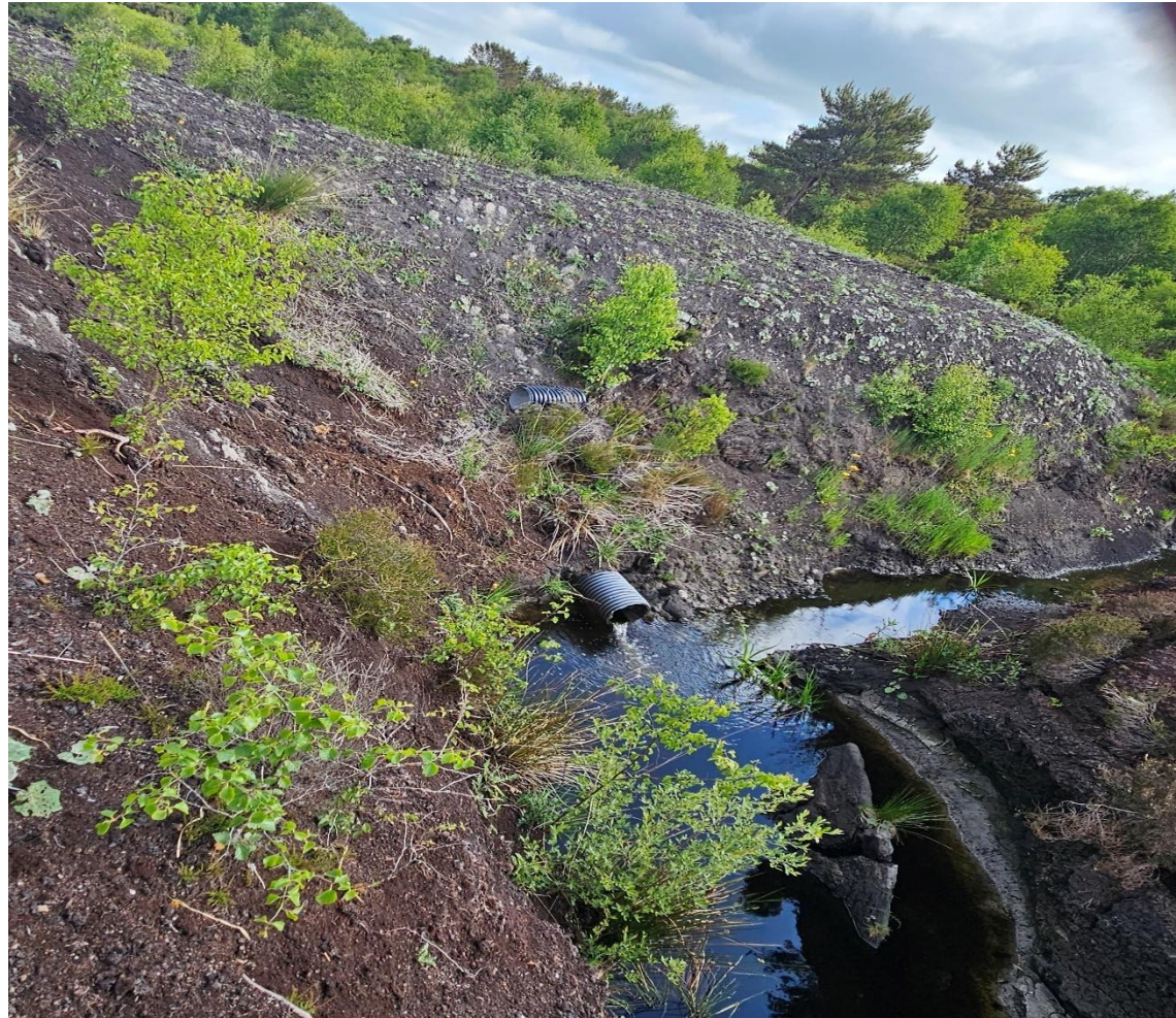
Photo 6: Discharge noted from one of the sediment ponds on the Eastern boundary.
