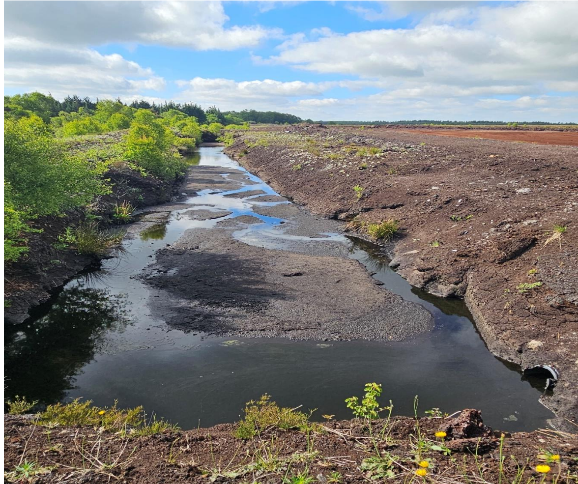
Photo 5: Heavy sedimentation noted in one of the sediment ponds at the Eastern boundary.
