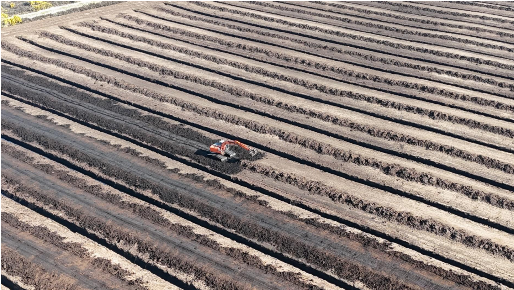
Photo 2: Excavator carrying out levelling works on the peatland.
