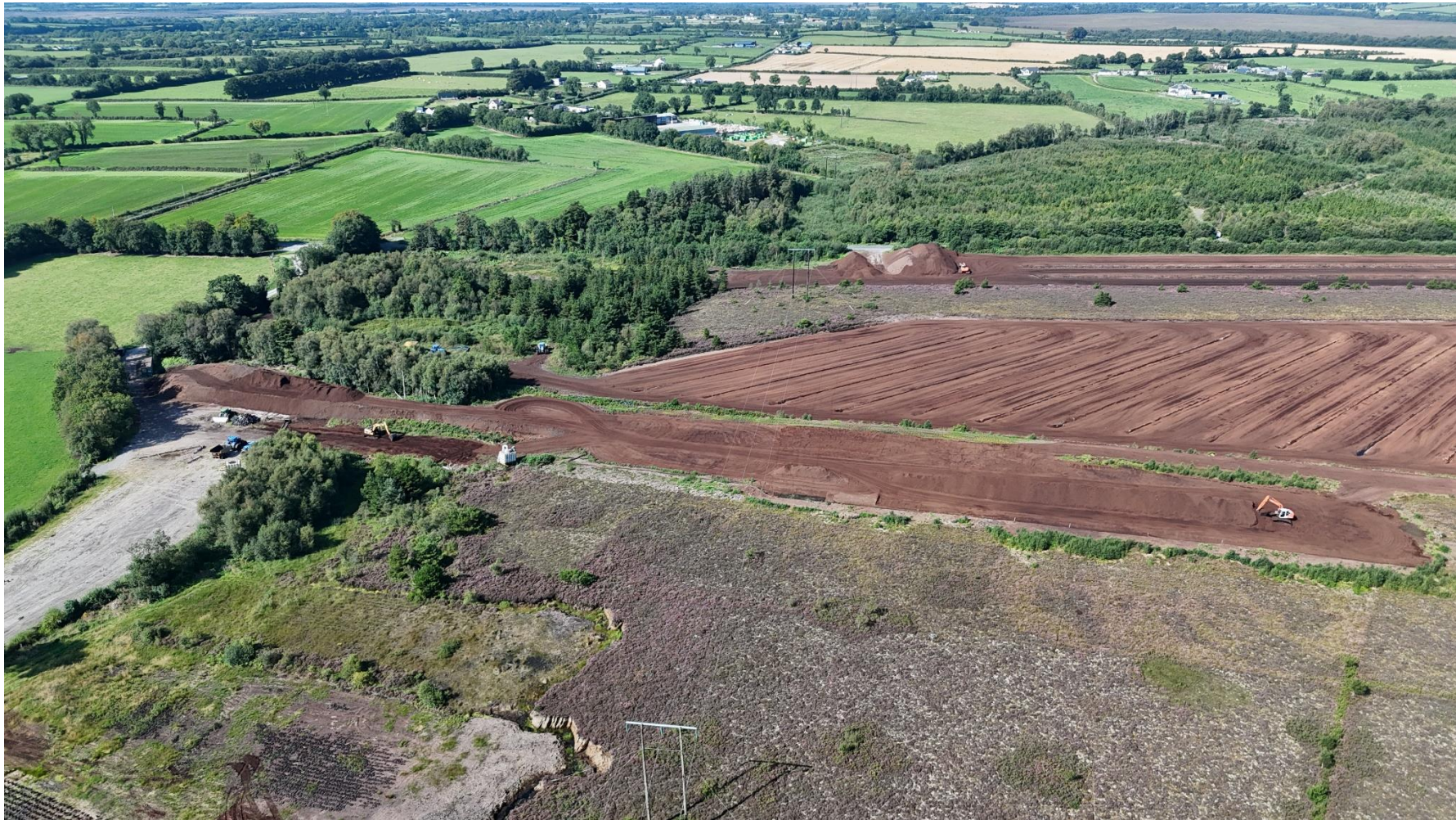
Photo 5: Stockpiles of milled peat noted at the south western part of the peatland, note excavators at a number of locations.
