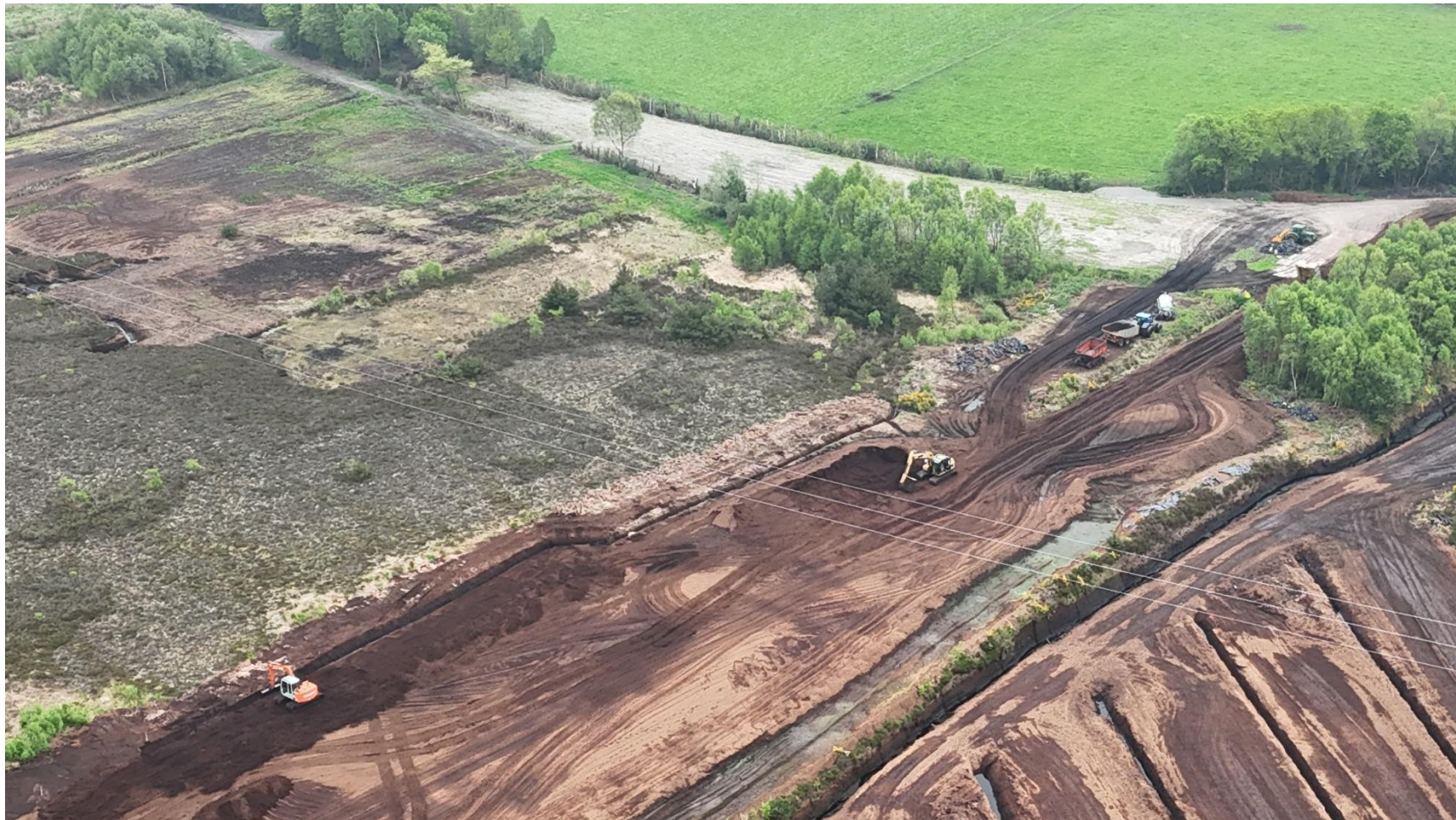
Photo 3: Drainage works noted to be ongoing and remaining milled peat stockpile noted at the southern part of the peatland.
