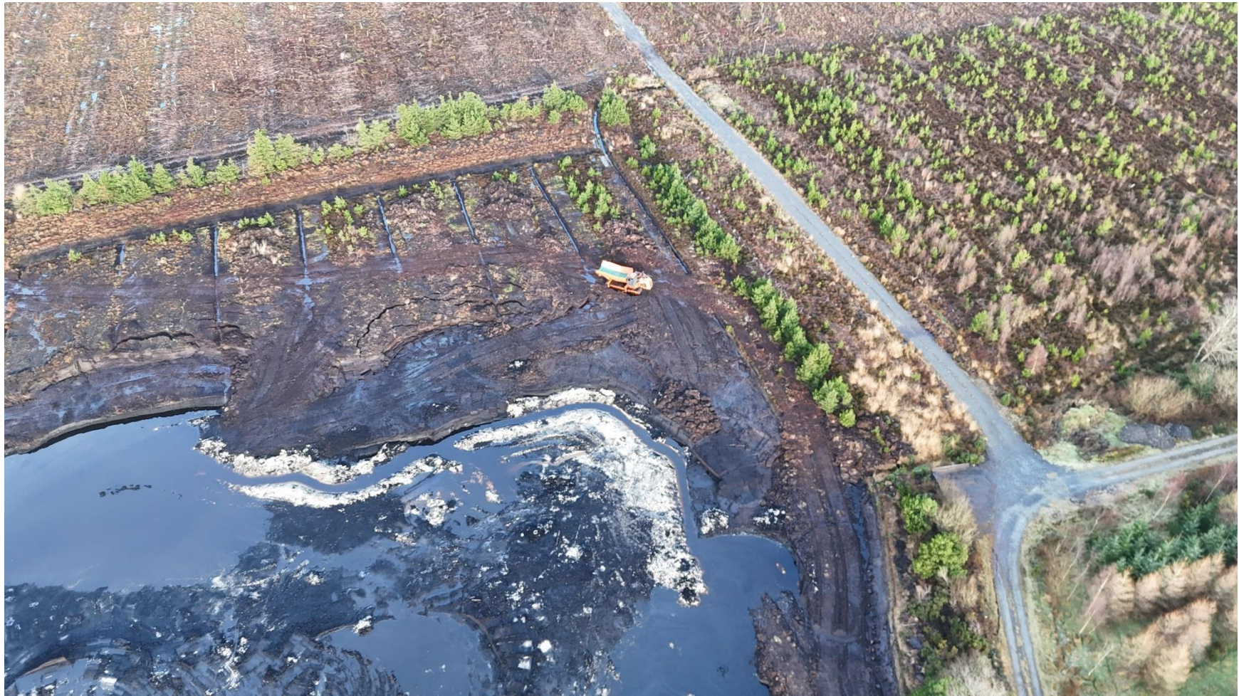
Photo 4: Photo of excavation area where peat had been excavated down to the marl.
