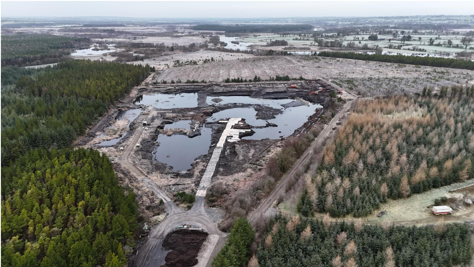
Photo 1: General overview of the peat extraction area showing peat excavation, road network and loading area.
