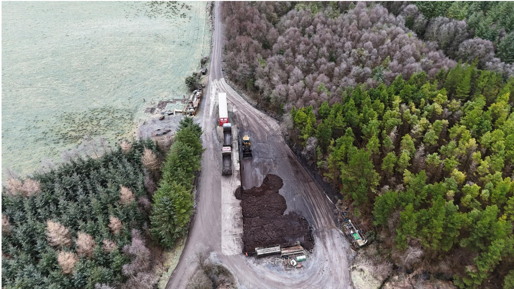
Photo 4: Significant quantity of peat noted at the loading area where peat is loaded on to lorries for transport off-site.
