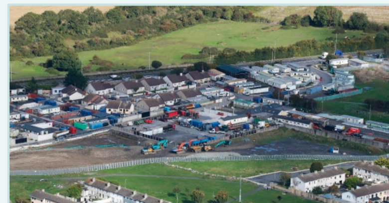
Aerial photo of the site following removal of waste mound (September 2025)
