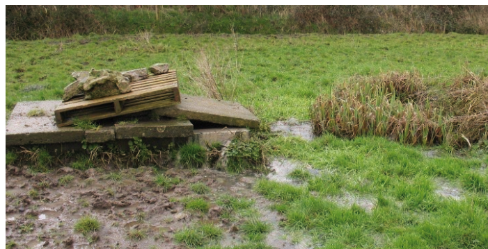
FIGURE 1: Ponding caused by a failed septic tank.
