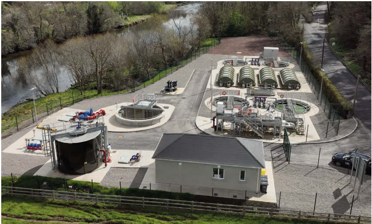
Figure 12: New waste water treatment plant at Innishannon, Co. Cork
