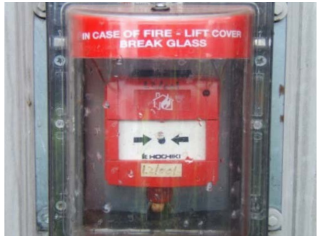
Figure 3.2 Break-glass unit
