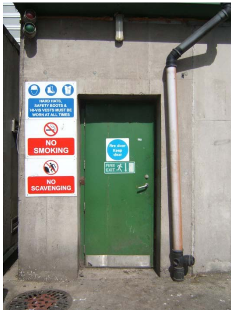
Figure 5.1 Fire exit free of obstruction
