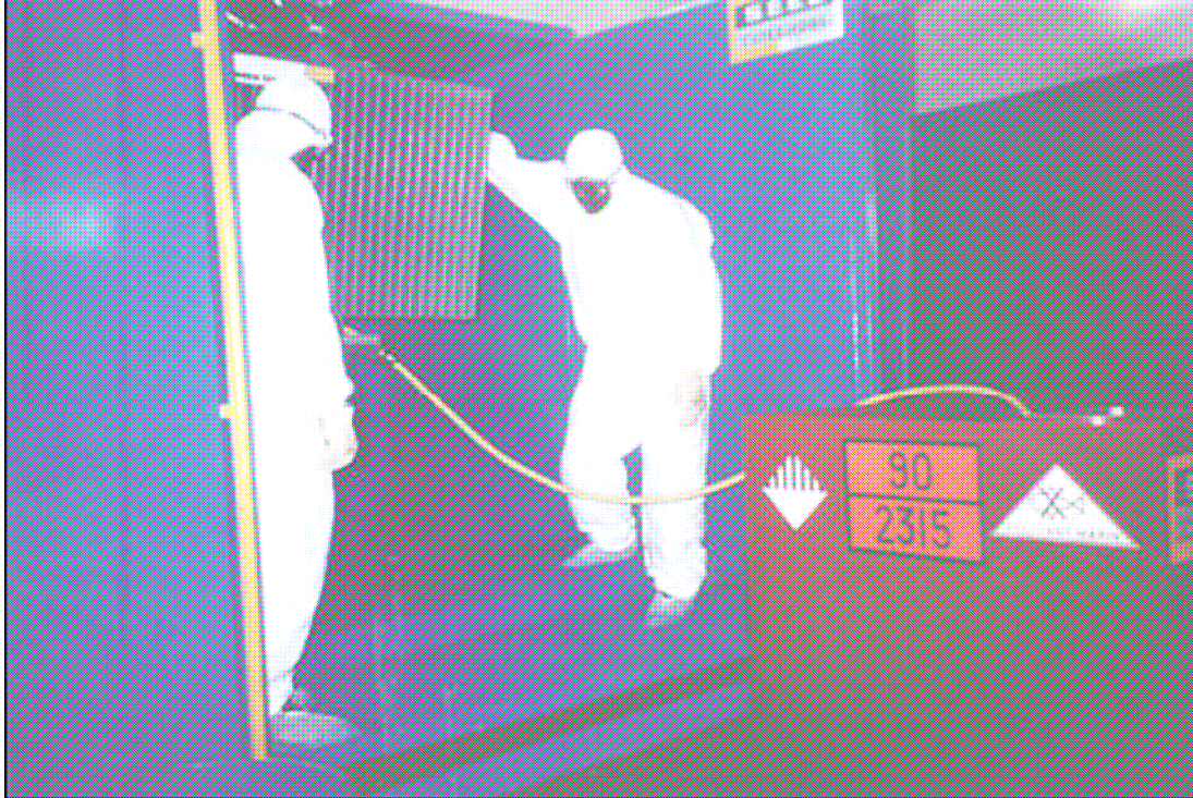
Photograph 1 – Decontamination of a Transformer 18
