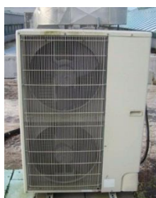
Figure 1: Split AC (Outdoor) Unit
