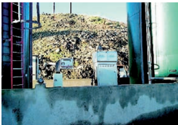
Figure 3.4. Bunded fuel oil tanks (Arkil Ltd, Rathangan, Co. Kildare).
