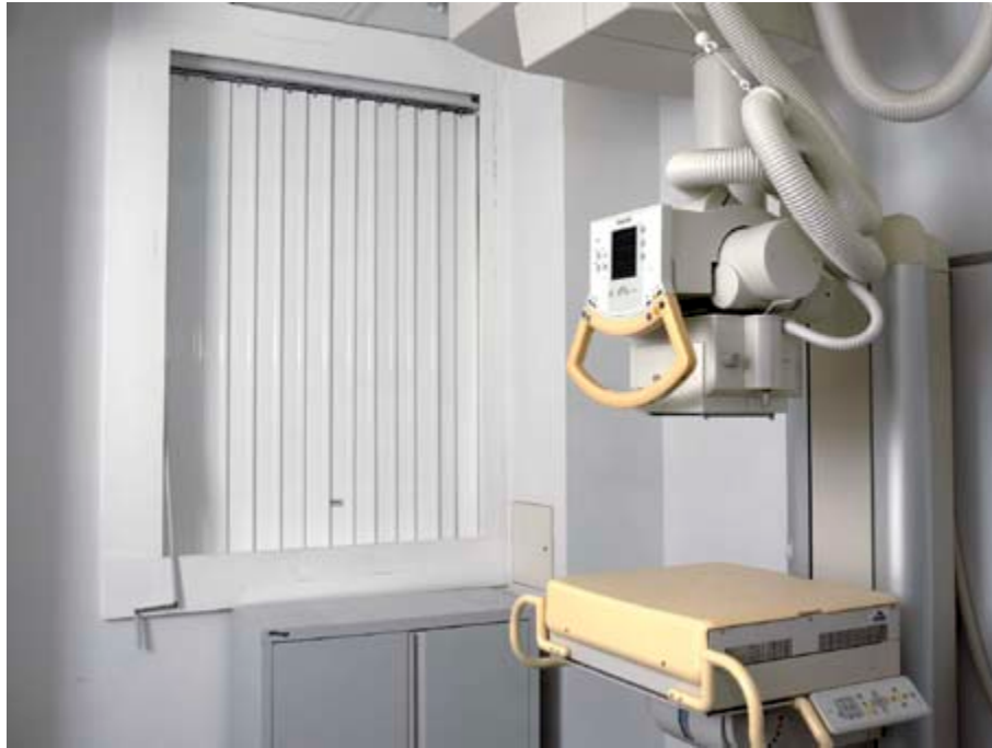
Photo 6.4 Lead blinds protecting windows
