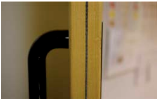
Photo 6.3(a) Lead doors
