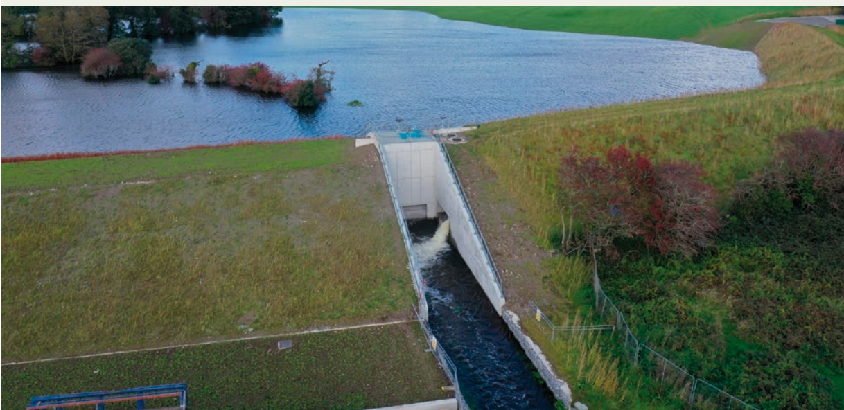
Figure 4.13 Clonakilty flood relief scheme – retention infrastructure
