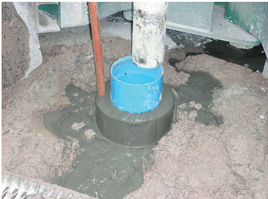
Grouting 6-inch PVC casing in place
