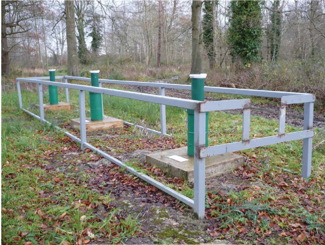
Completed well cluster at Ryewater with data loggers installed
