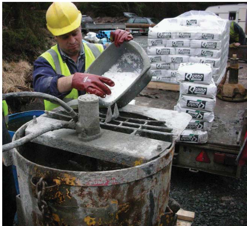
Adding calcium chloride to grout batch plant
