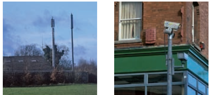
Figure 4.1 Photos of mobile phone mast and microcell-antennas.
