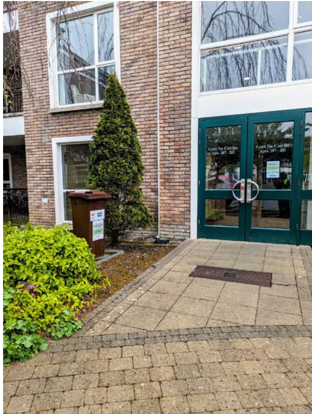
Figure A6.3. Phase 2 food waste bin at entrance trial. For the duration of this trial and its extended period in the summer months of 2024, the food waste bin was placed in this location proximal to the apartment entrance door.
