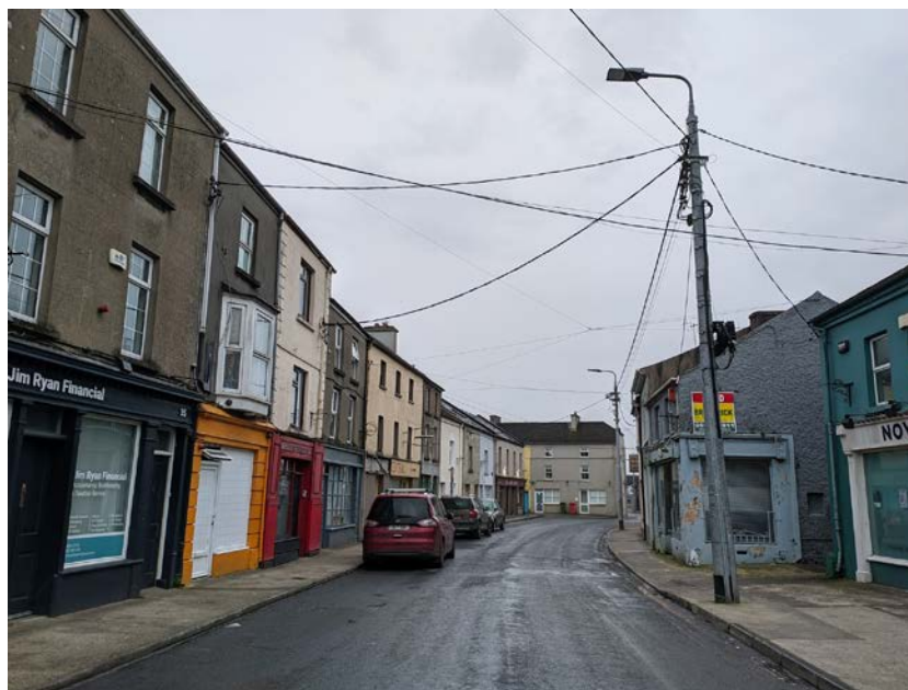
Figure 2.13. Set piece of urban vacancy, which forms part of a cluster of 21 vacant and 3 derelict buildings in the town centre of Thurles, Co. Tipperary, on Croke Street, March 2024. Credit: Liam Heaphy.
