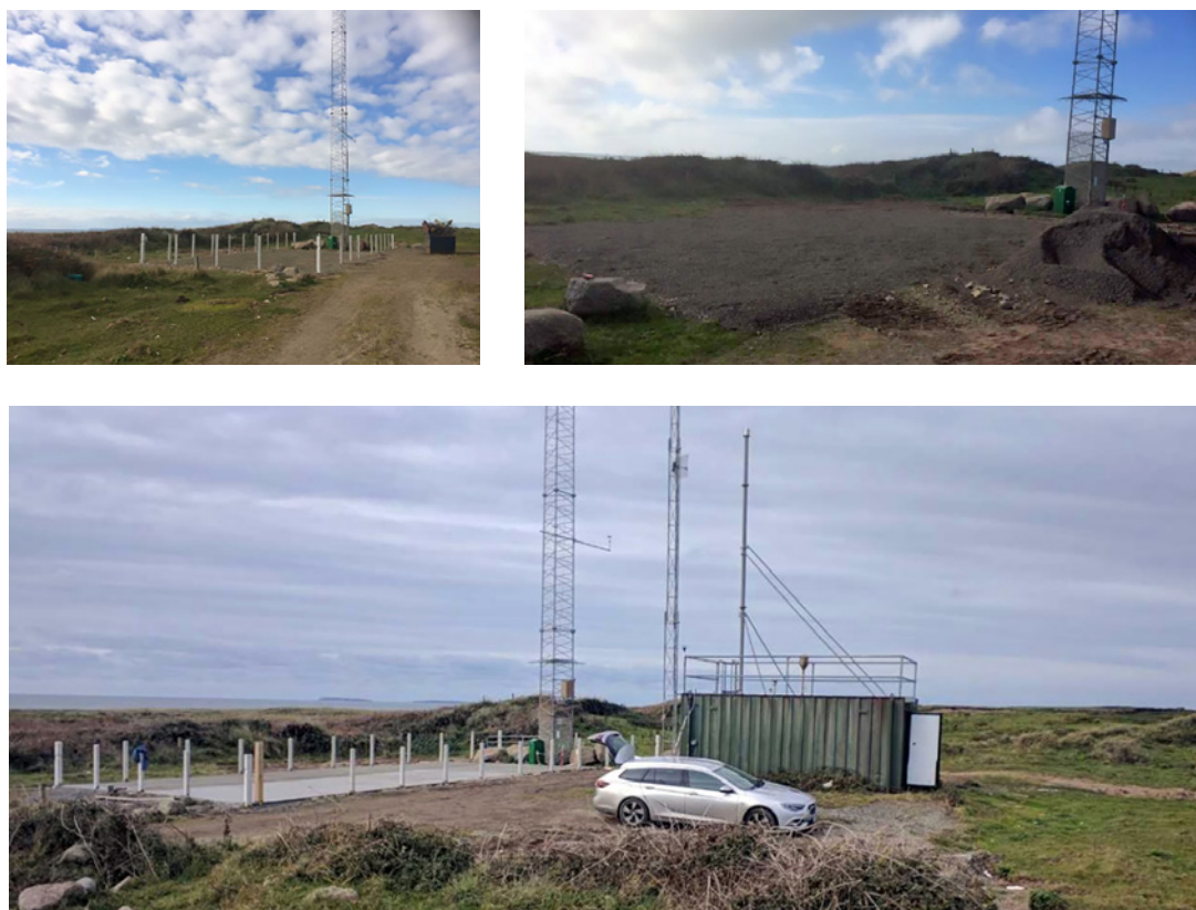
Figure 5.2. Start of site redevelopment at Carnsore Point.
