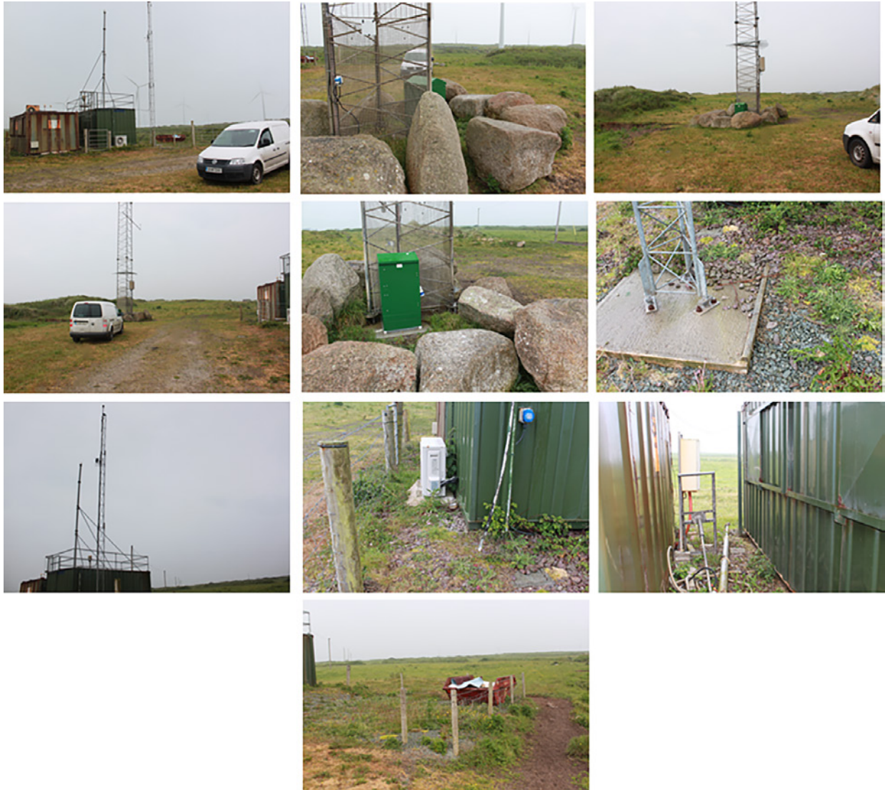
Figure 3.3. Current Carnsore Point infrastructure.
