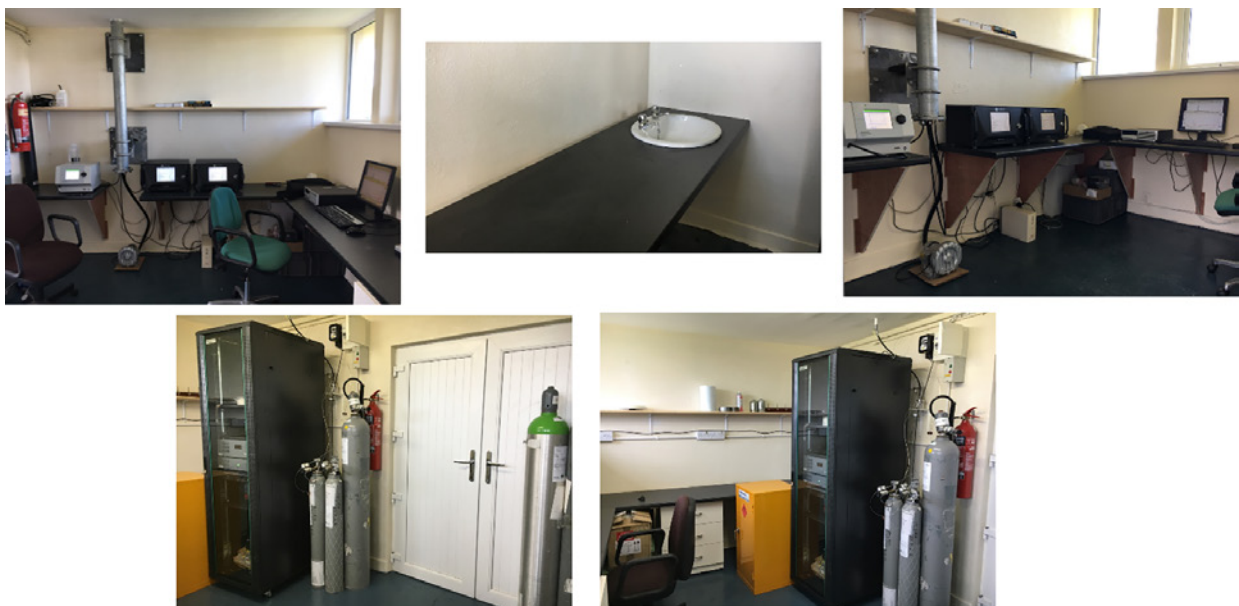
Figure 3.4. Refurbishment of the laboratory at Malin Head.
