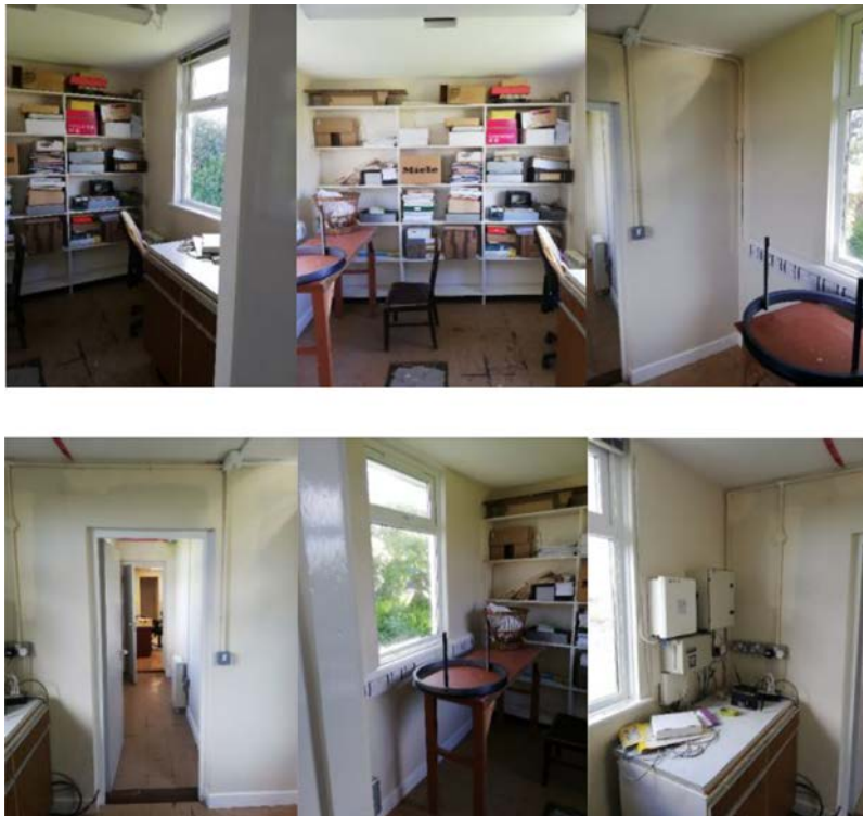
Figure 2.5. Disused room in top cottage before refurbishment.
