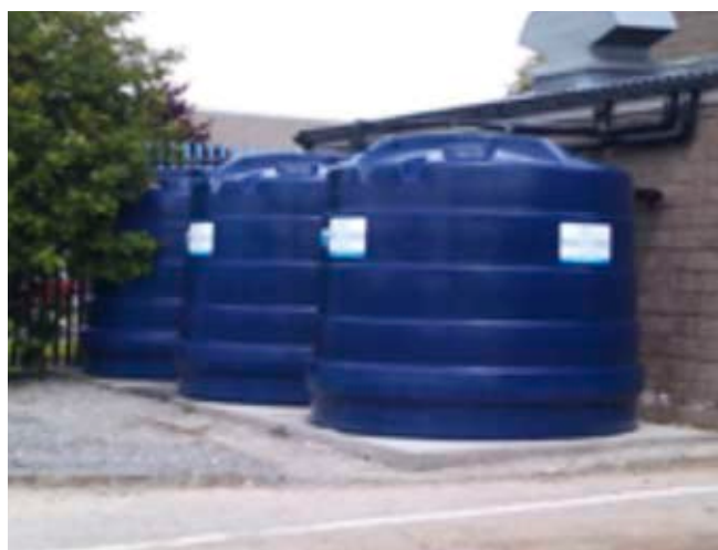
Rainwater harvesting installation at OLM
