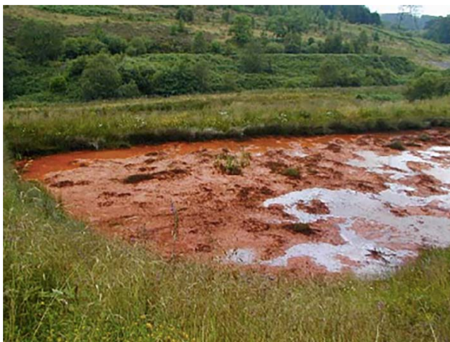
Figure 6.1. Accumulation of iron oxide and hydroxide on the surface of a RAPS. Reproduced from Wiseman (2002). Contains Environment Agency information. © Environment Agency and database right.
