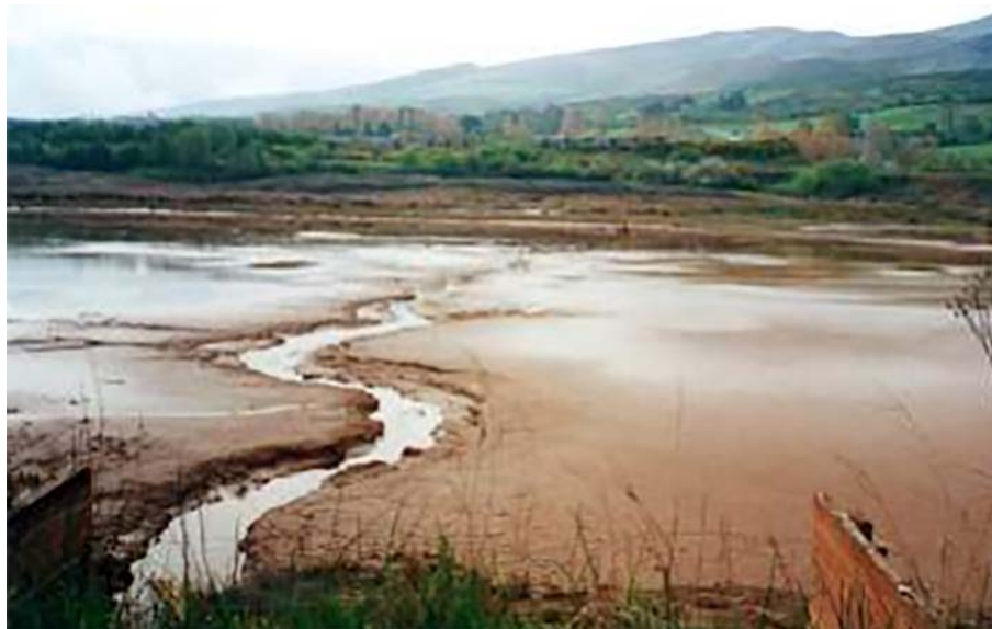
Figure 2.1. Surface water ponding on tailings at the Silvermines site.
