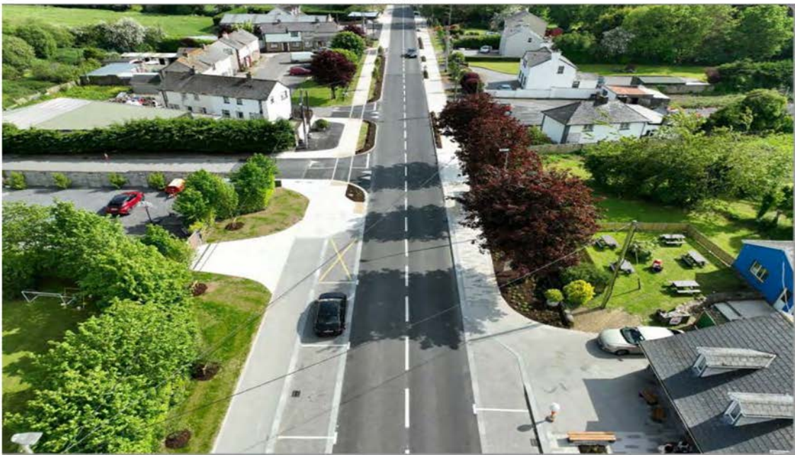
Figure 6.2. Example of TII soft-landscaping redevelopment of a bus stop in Grangemockler, County Tipperary. Photos courtesy of TII.
