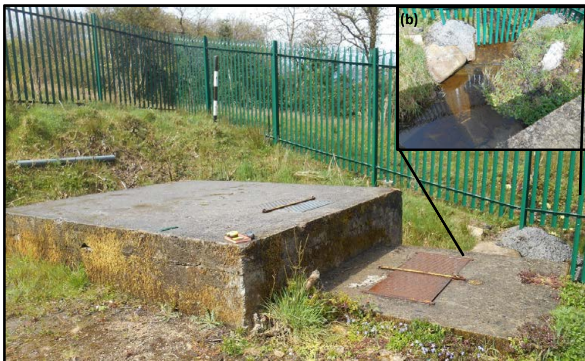
Figure G3.24. Swanlinbar P.W.S. showing the (a) spring chamber and (b) unpiped spring overflow.
