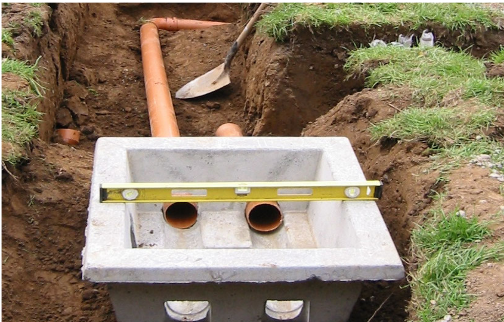
Figure 3.6 Installation of distribution box and connecting pipes.
