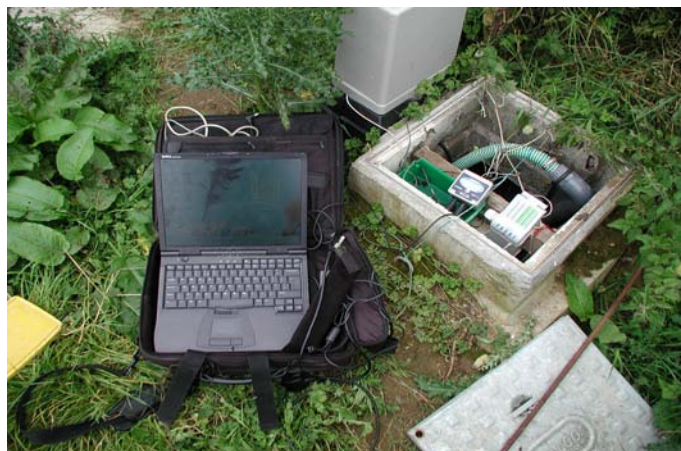
Figure 4.4 Easylog ultrasonic level detector on Site 2.
