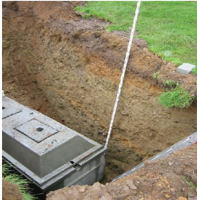
Figure 2.8 Trial Hole on Site 3.
