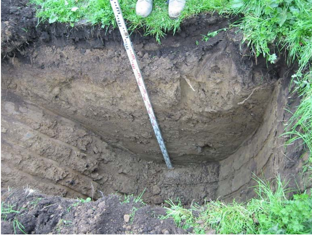
Figure 2.6 Trial hole on Site 1.
