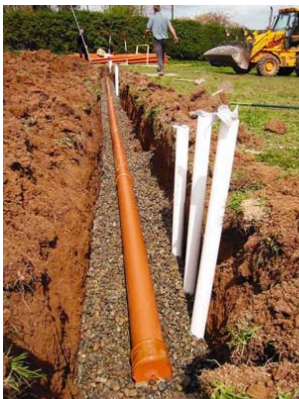
Figure 3.3. Construction of percolation trench.
