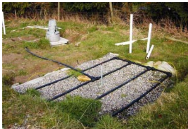
Figure 3.7. Completed stratified sand filter on Site 4.
