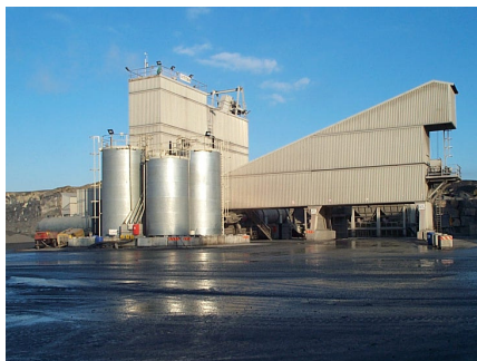
Energy efficient asphalt plant incorporating insulated bitumen tanks and aggregate bins (Roadstone Provinces Ltd., Bunratty, Co. Clare)
