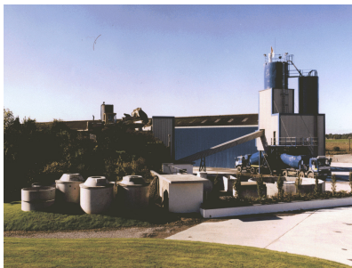
Concrete batching plant (Shay Murtagh Ltd., Raharney, Co. Westmeath)
