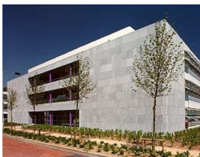
Use of dimension stone at East Point Business Pk. (Feelystone Ltd., Co. Kilkenny)
