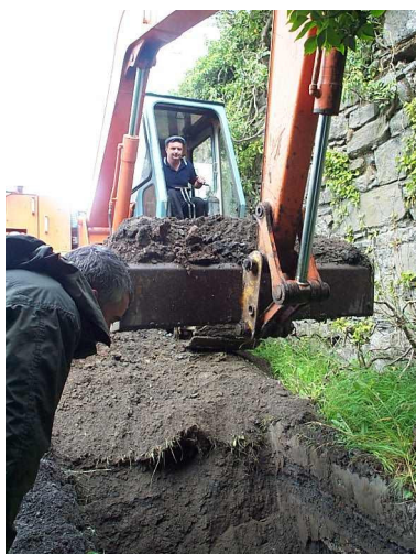
Trial excavation under supervision of licensed archaeologist (Harrington Concrete (Sligo) Ltd., Ballysadare, Co. Sligo)
