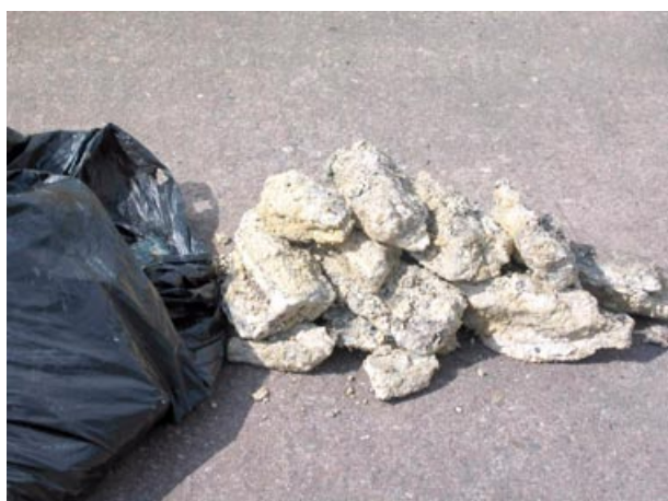
Figure 6.1: Solidified Fat Pieces Removed from Ballincollig Sewer System in Co. Cork
