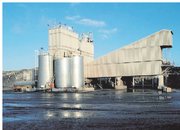
Figure 4.4. Energy-efficient asphalt plant incorporating insulated bitumen tanks and aggregate bins (Roadstone Provinces Ltd, Bunratty, Co. Clare).
