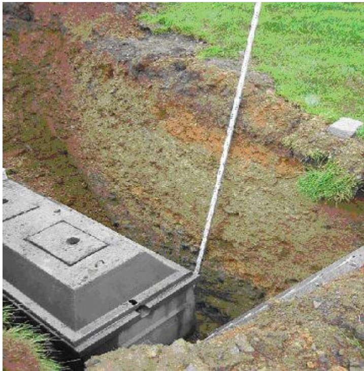
Figure 3.3 Trial Hole on Site 3.
