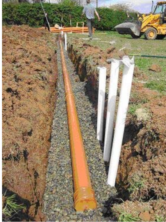
Figure 3.8 Percolation pipe on 250mm gravel bed.
