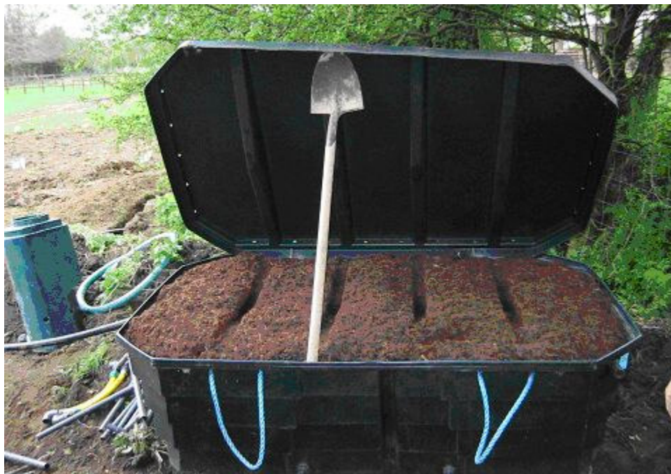
Figure 3.5 Open Puraflo ® module containing fibrous peat media.
