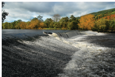
Inniscarra weir, River Lee, Co. Cork (adjacent to EPA office Cork)
