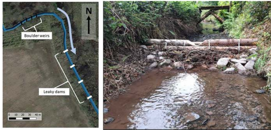
Figure 2.6. LDs at Site 2. The left panel shows the LDs' location and the basic design. The right panel shows the view from the upstream side of the first LD, showing woody debris build-up following the first high-flow event following installation (June 2022).
