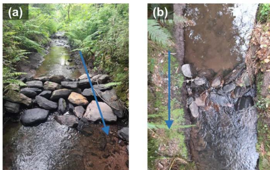
Figure 3.2. Instream weirs during (a) low and (b) medium flows. Blue arrows indicate direction of flow. Panel (a) shows the downstream side of a low-head boulder weir (foreground) and the next most upstream weir (photo taken on 26 May 2022). Panel (b) shows the view looking down at a boulder weir and streambed (photo taken on 4 April 2022). Sediment accumulation and slow-moving water are visible at the upstream side, and a clear streambed and high flow are visible on the downstream side.
