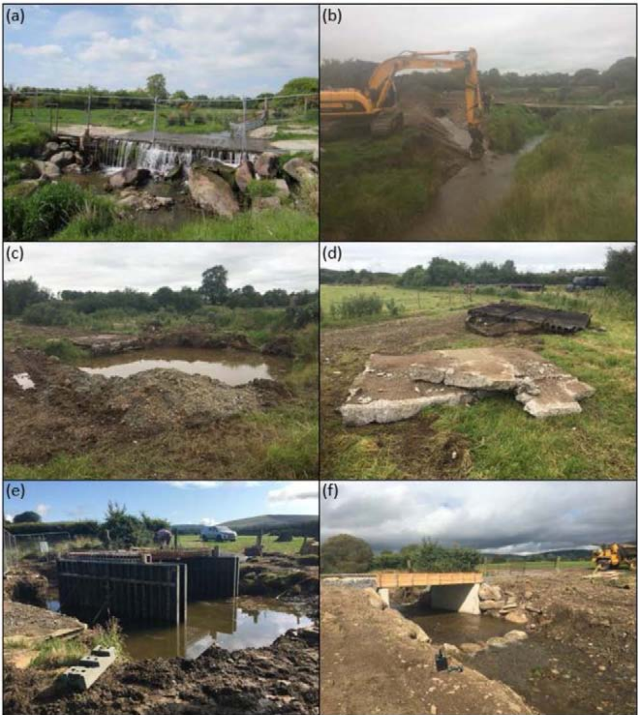
Figure 2.5. Restoration phases on the Browns Beck Stream: (a) before the ford removal, (b) creation of a diversion channel (October 2018) and (c and d) removal of the concrete ford structure (July 2019), (e and f) installation of the culvert (August 2019).
