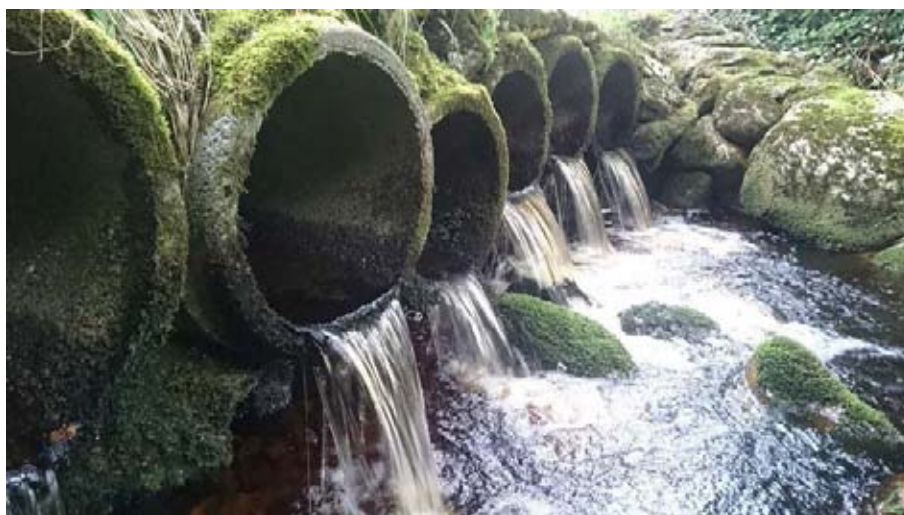
Figure 10.1. Culverting that would impact fish movement.
