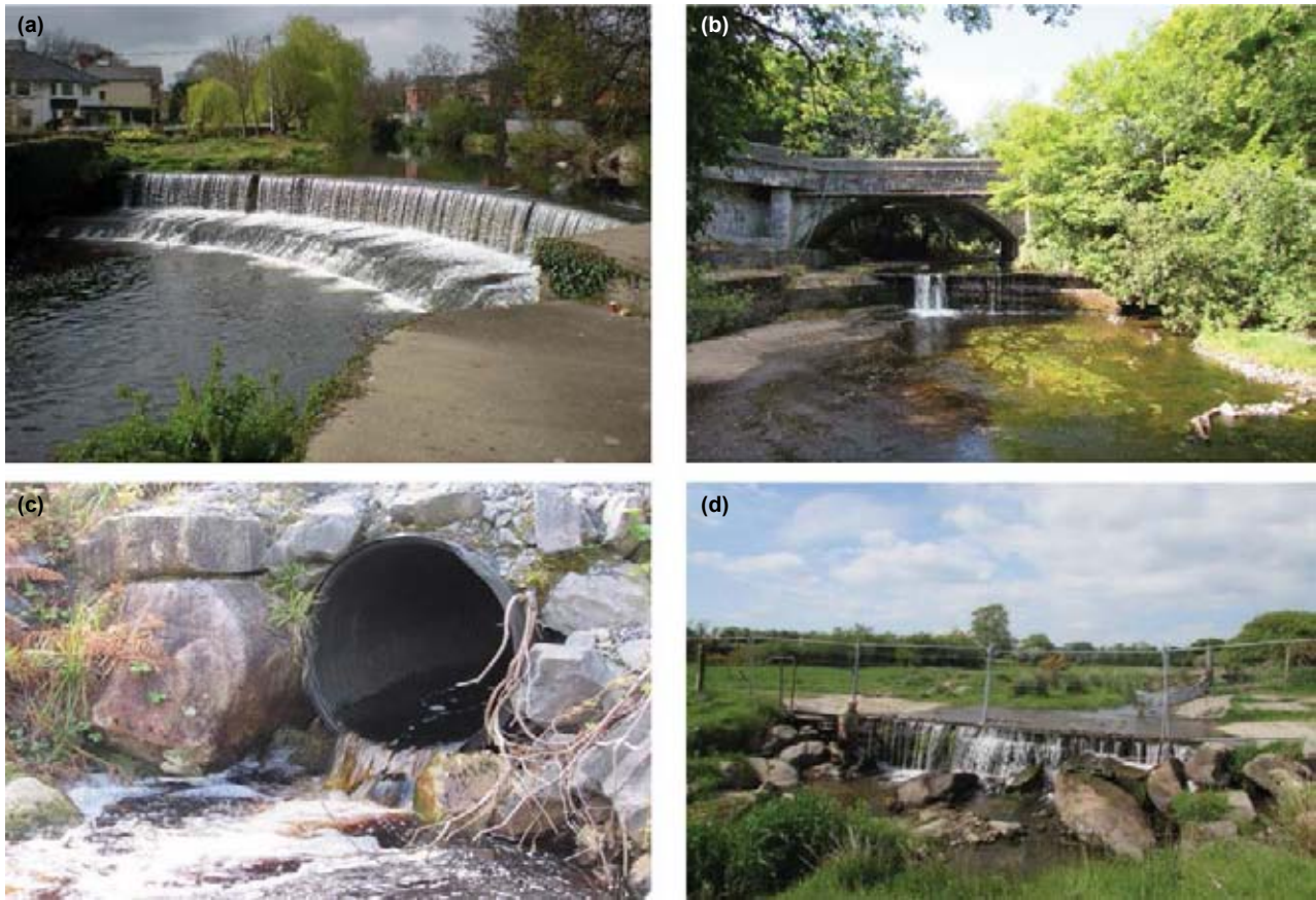
Figure 1.1. Four broad categories of low-head barriers on Irish rivers. (a) Weir on the River Dodder, Dublin city; (b) bridge apron on the River Dodder, Dublin city; (c) culvert on the River Owenboliska, Co. Galway; and (d) ford on Browns Beck Brook, Co. Wicklow.
