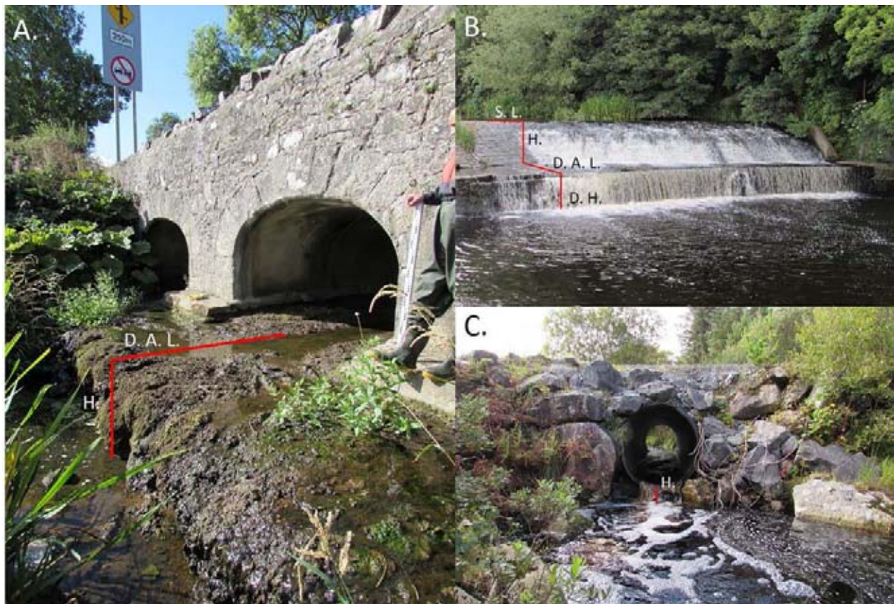
Figure 3.3. Photographs showing varying barrier types and some of the physical measurements recorded. (A). Bridge apron with a drop (H) at the downstream end of the apron (D. A. L.). (B) Sloping weir (S.L. and H) with a downstream apron (D.A.L.) and a downstream drop (D.H.). (C) Culvert with a drop (H). D.A.L., length of apron; D.H., height of drop; H, height; S.L., sill length measured on the horizontal. Reproduced from Atkinson et al. (2020); licensed under CC BY 4.0 ( https://creativecommons.org/licenses/by/4.0/ ).
