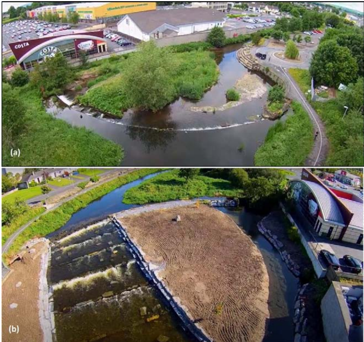
Figure 2.7. Hanover Weir (a) viewed downstream on River Burren prior to remedial works and (b) viewed downstream following the construction of the rock ramp fish pass. Images: Inland Fisheries Ireland.
