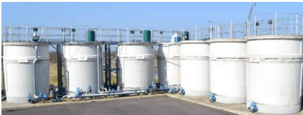
Figure 3.6. Photograph of the field-scale pumped flow biofilm reactor at the Water Research Facility
